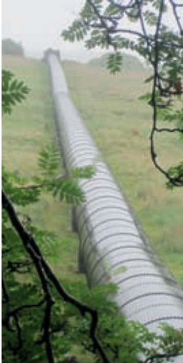
A McArdle hazard to crawl under.
