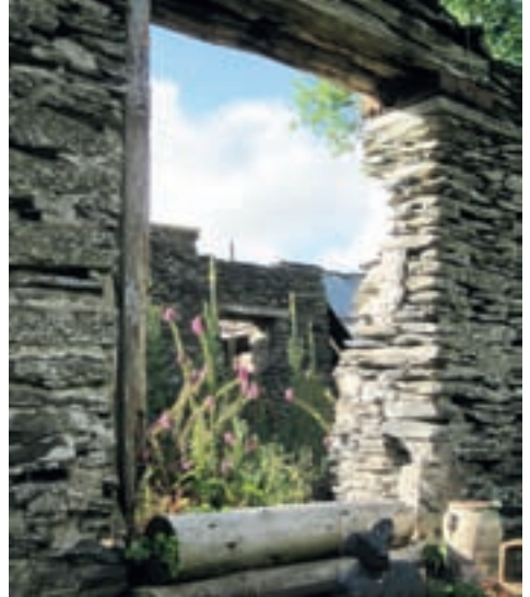
Meri has repaired the house, some outbuildings still to do.
