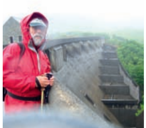
Crossing the dam of the Trawsfynydd Reservoir.
